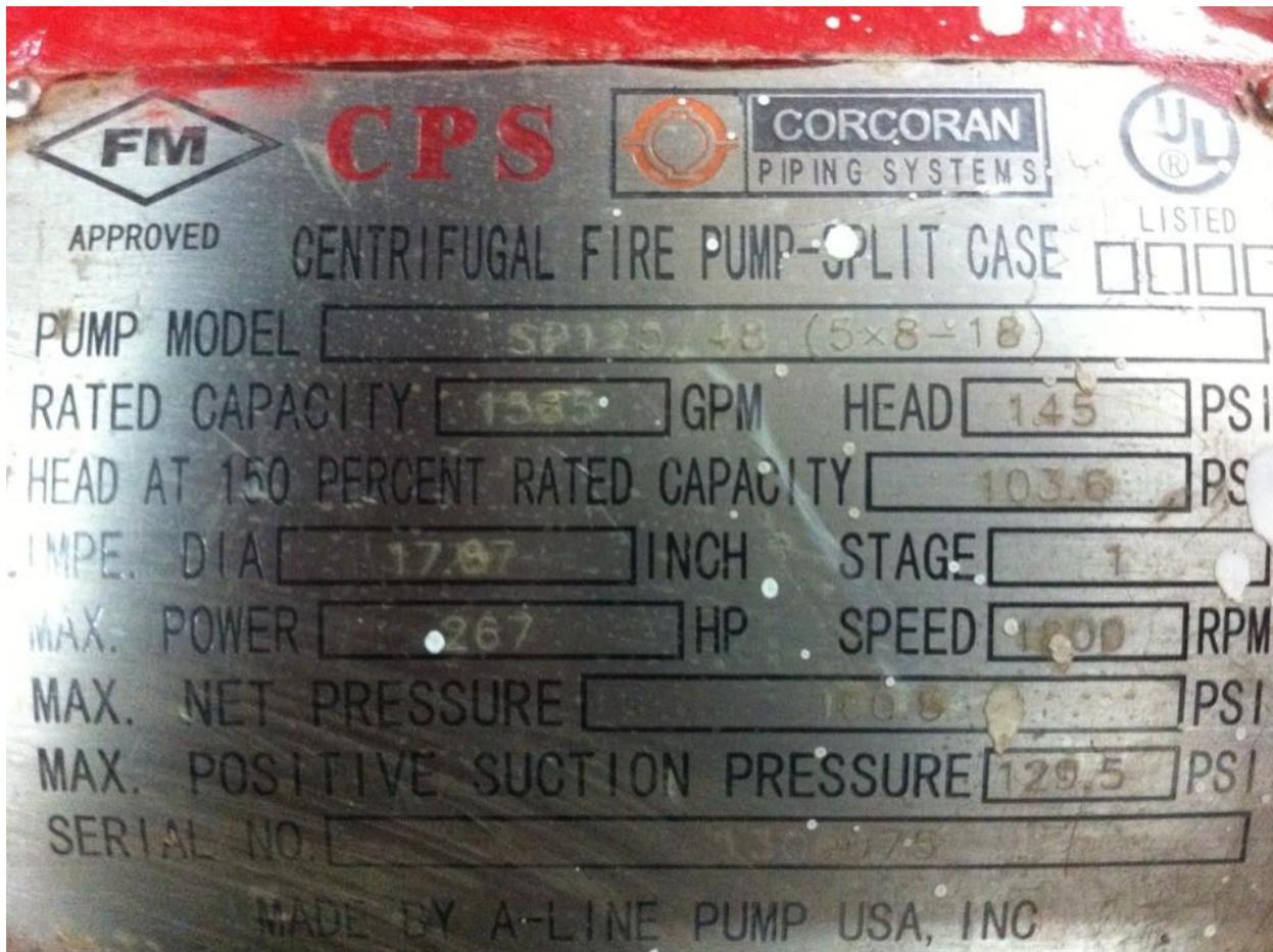
Figure 1. CPS Counterfeit Nameplate [Close up view]
