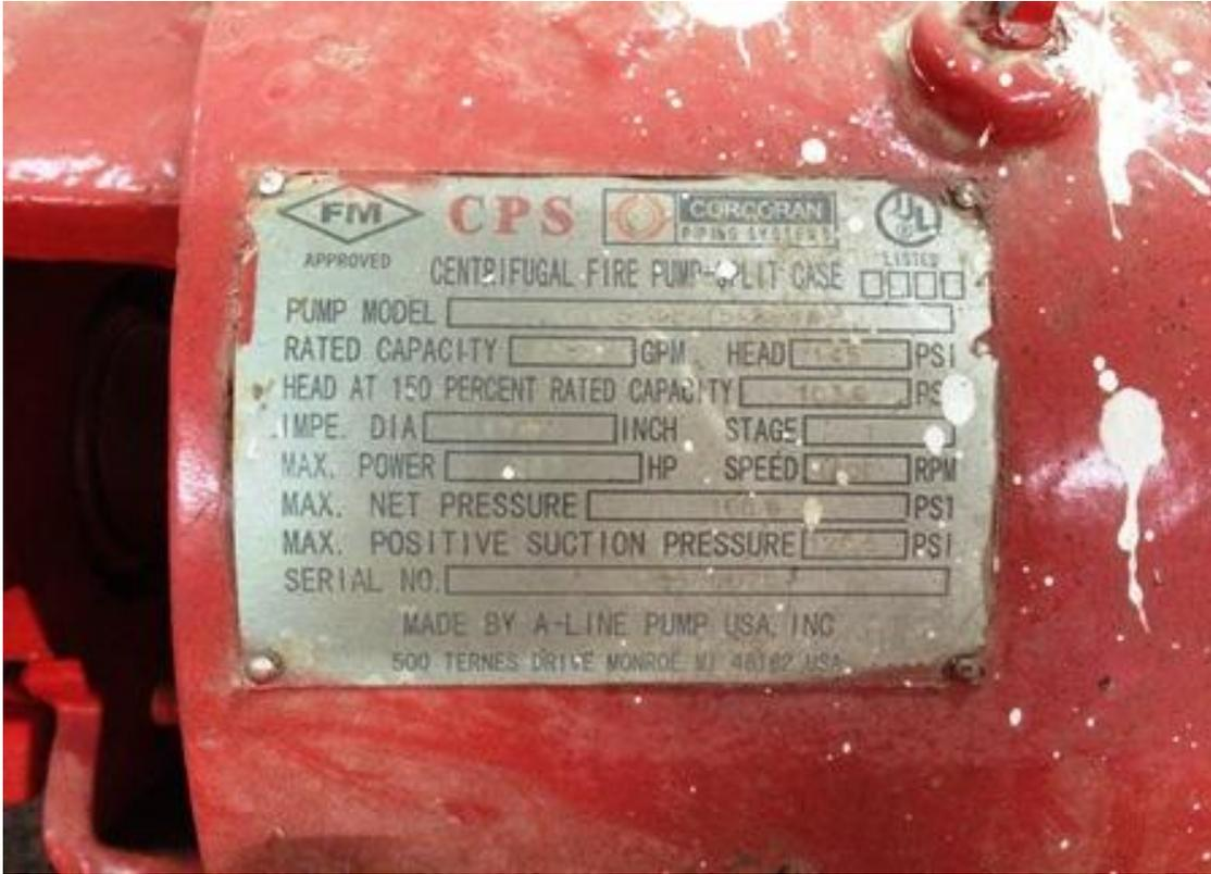
Figure 2. CPS Counterfeit Nameplate
