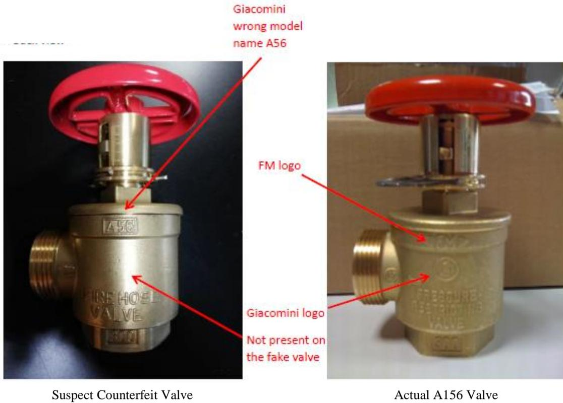
**Figure 2 – Model A156 Valves:** The suspect counterfeit valve has the wrong model number cast on to the valve body and it is missing the Giacomini logo.
