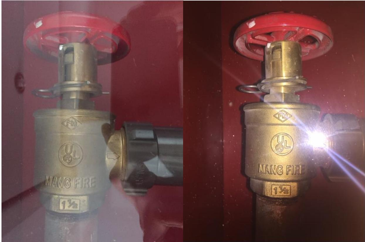
**Figure 1 – Suspected Counterfeit Pressure Reducing Valves**
