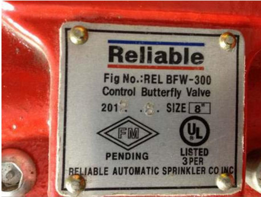
**Figure 1.** Nameplate of Reliable Automatic Sprinkler Co. Model REL-BFW-300 size 8 inch NPS bearing an “FM Approval – Pending” mark
