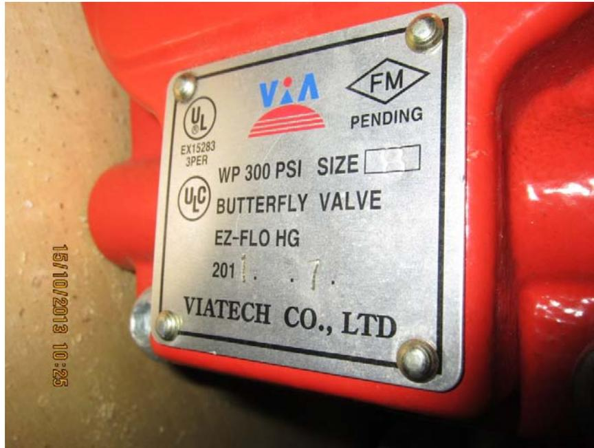
**Figure 1.** Nameplate of VIA Tech Model EZ-FLO HG size 8 inch NPS bearing an “FM Approval – Pending” mark
