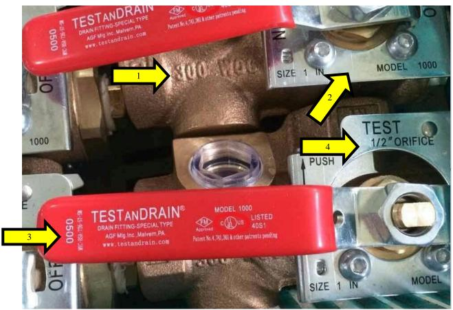
Figure 1 – Counterfeit Model 1000 Valves
