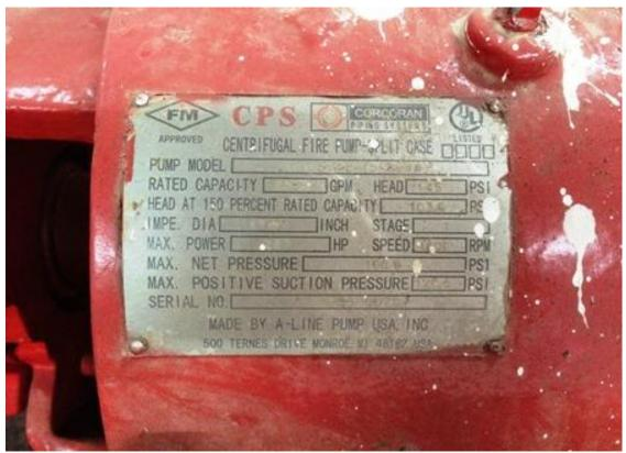
Figure 2. CPS Counterfeit Nameplate
