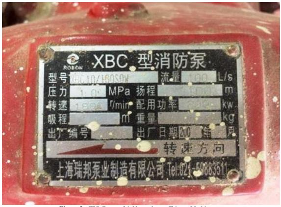
Figure 3. CPS Counterfeit Nameplate – Chinese Markings
