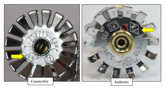
**Figure 5.** Counterfeit FM Approvals mark on the pendent style sprinkler (left) and the authentic FM Approvals mark on an authentic Globe GL5651 sprinkler (right).
